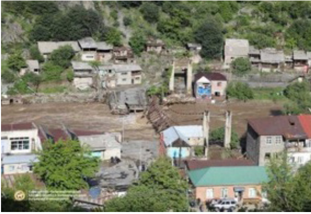
Image 12. Destruction of the bridge at Sanahin
