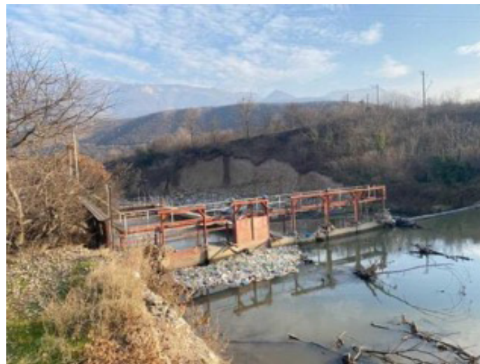
Image 29. Dam upstream of Khashtarak bridge
