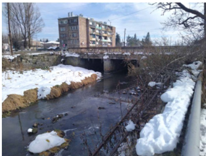
Image 5. Tashir river with accumulations in the river bed
