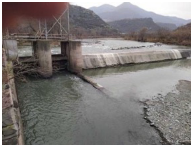
Image 32. Dam at the Shnogh reservoir
