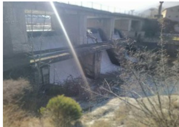
Image 28. Dam at the Ijevan reservoir
