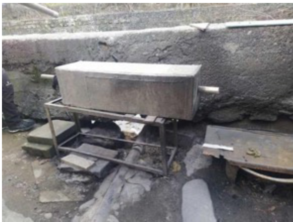
Image 8. Another hole in the wall
