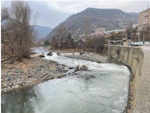
Image 25. Remains of a dam diverting water to the protection wall
