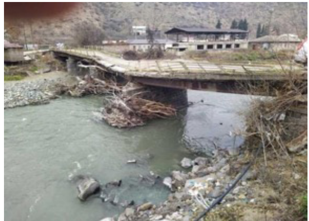
Image 17. Ayrum bridge in December 2024
