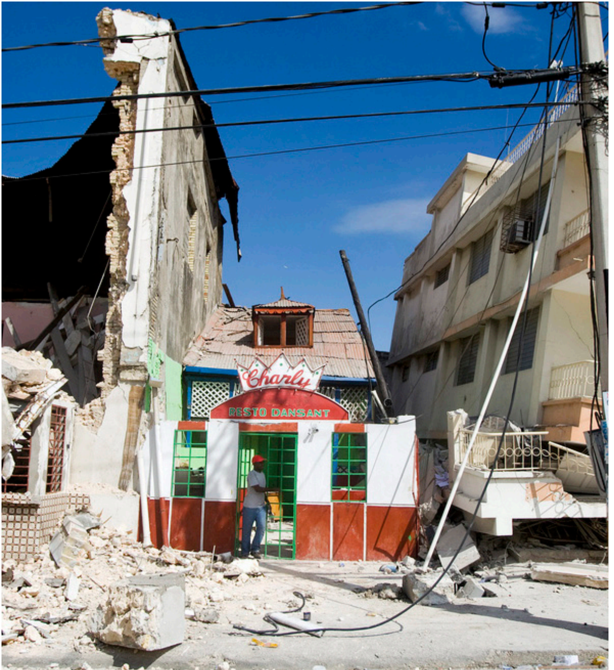
Port-au-Prince, Haiti, 2010: It is not the earthquakes that kill people, but the buildings collapsing on them.
