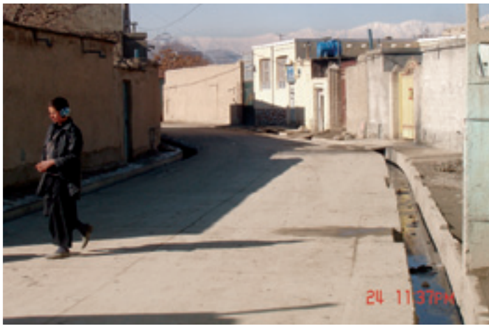
Kabul Municipality, Afghanistan: before and after urban improvement works with drains and sanitation.
